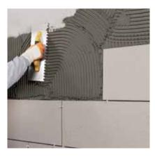
According to the size of the tiles, fix tiles with either single buttering method (the adhesive is buttered on the substrate) or double buttering method (for tile sizes > 33x33 cm, adhesive should be buttered onto the tile back as well). The tiles must be fixed within the open time of adhesive and pressed on with a twisting and sliding action to achieve a good contact.
