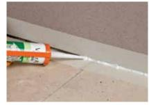
Expansion joints should have minimum width of 6-10 mm. Expansion joints should be insulated by using proper profiles or mastics. Cementitous grouting materials are not appropriate for expansion joints.
